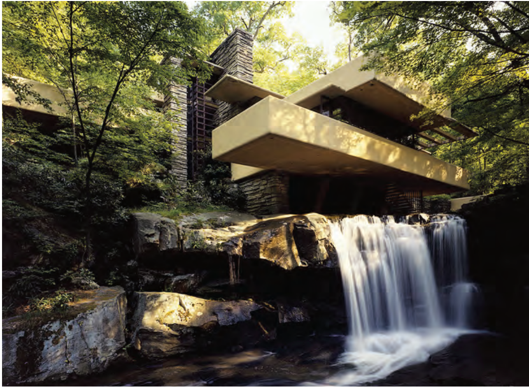
HERE: Fallingwater, classic view from the SW elevation courtesy of the Western Pennsylvania Conservancy
